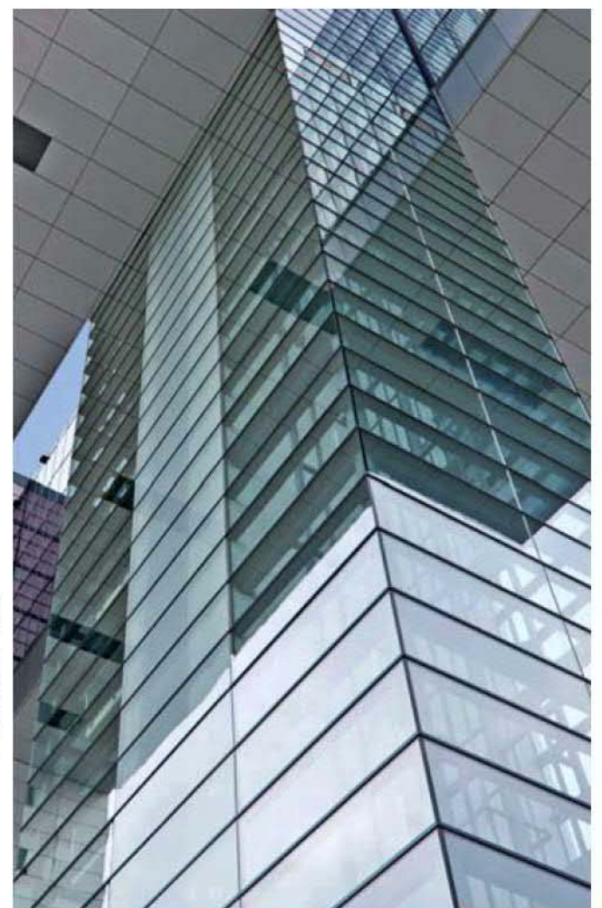
Glass lift tower
