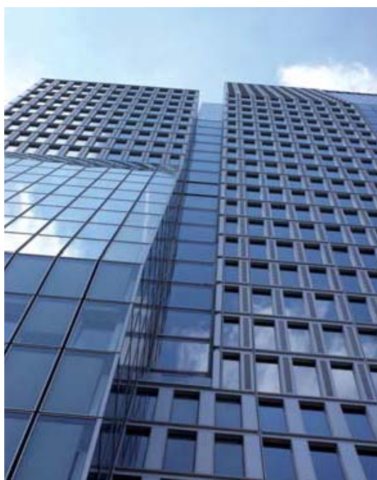
Details of double-skin facade, viewed from below
