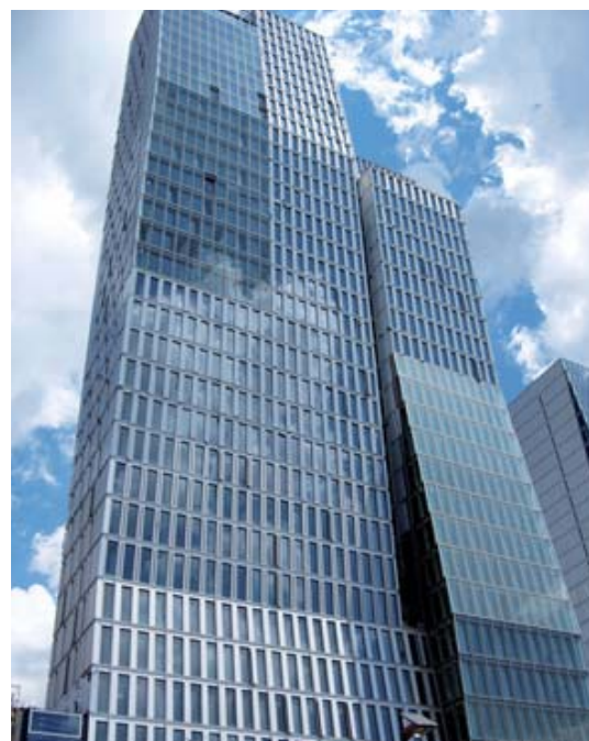
Eastern and western front of office tower with double-skin facade (left) and single-skin facade (right)
