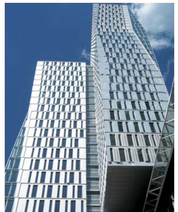
Eastern and western front of office tower with double-skin facade (left) and single-skin facade (right)
