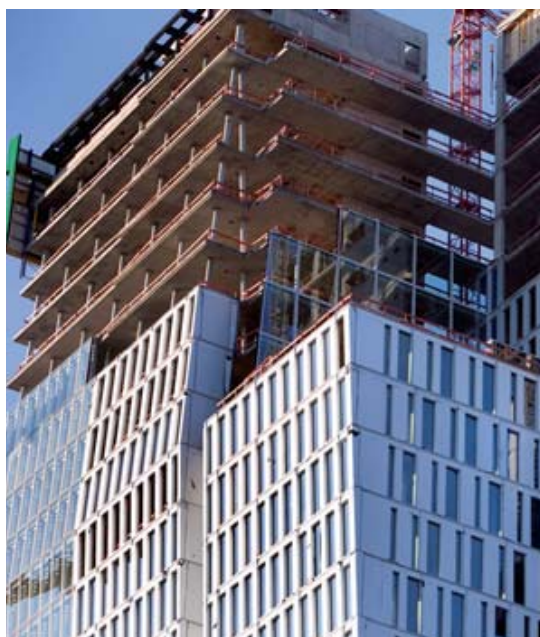
Office tower under construction and nearing completion ...
