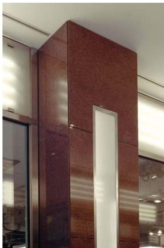
Stone cladding in shopping mall
