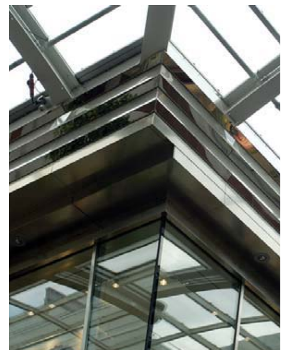
Junction of mall facade with glass roof
