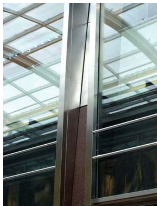
Shopping mall, curtain wall detail
