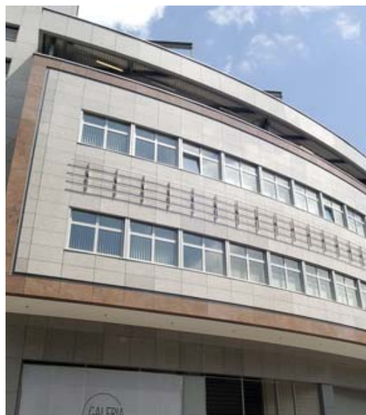
Shopping mall exterior
