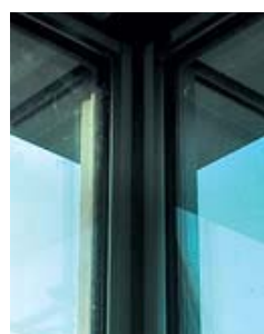
Connection of glass fin to reinforced-concrete slab
