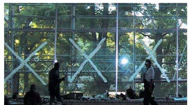
Installation of glass windows in first-floor multi-purpose space
