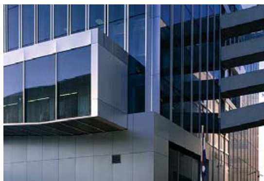
A projecting glazed ramp with glass flooring offers views of the street below
