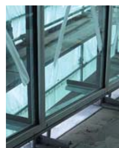
Glass fins used to stiffen facade assembly
