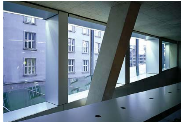
View of glass ramp from interior
