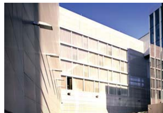
The main block is shielded by an L-shaped stone and concrete "paravent"
