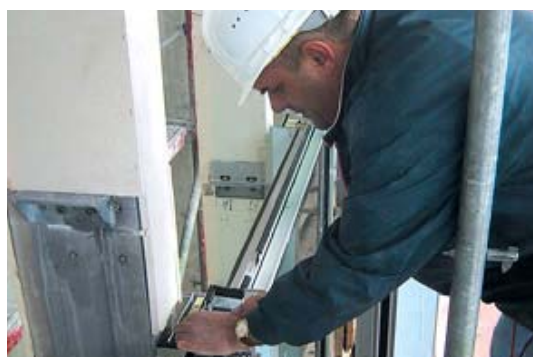
Sealing of horizontal coupling sections in shaft-box facade
