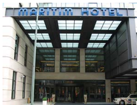
Canopy overhanging main entrance
