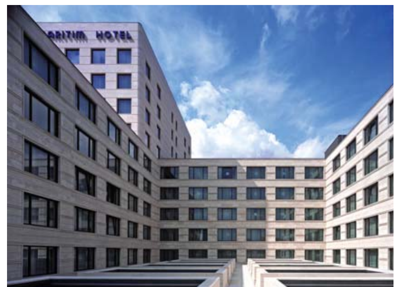
Rooftop courtyard over Small Ballroom
