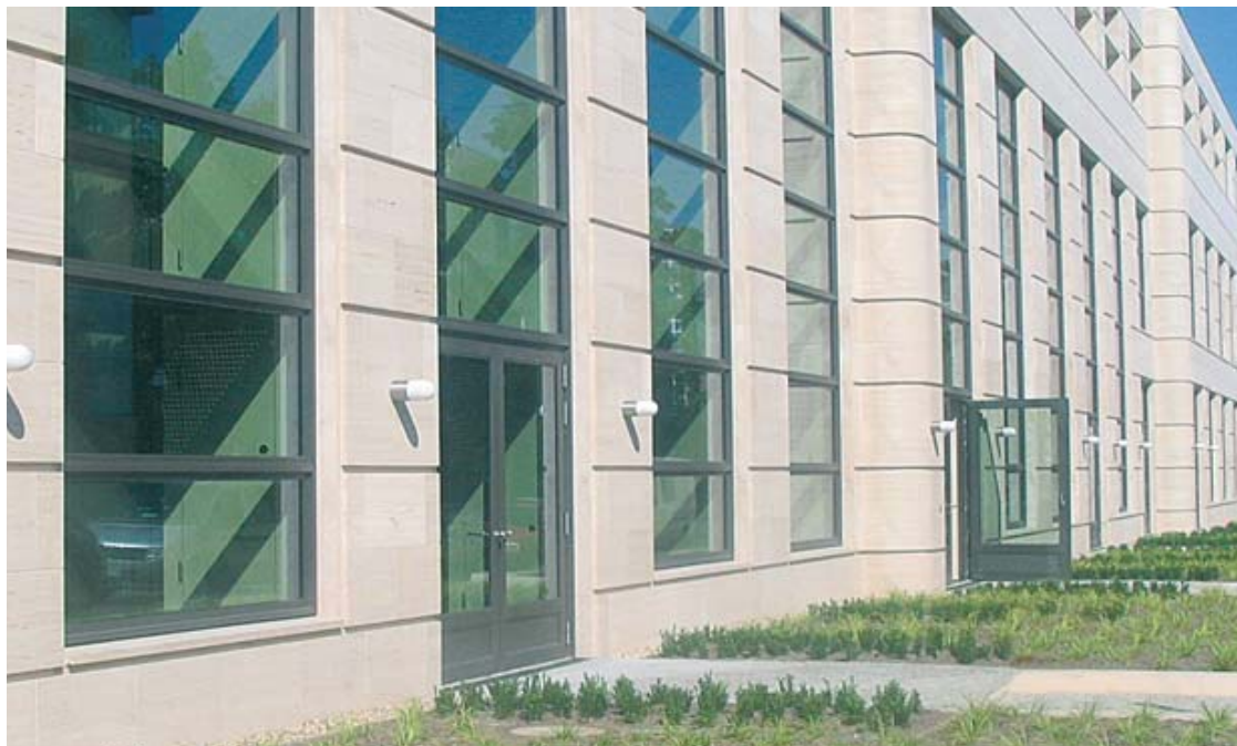
View along facade
