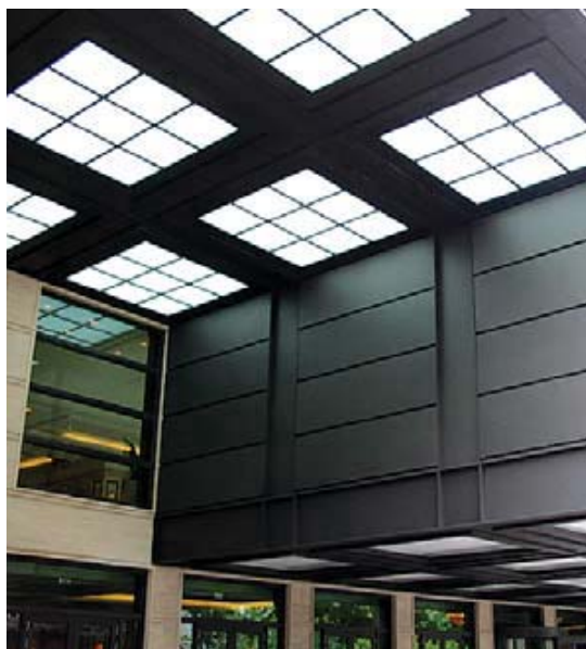
Canopy main entrance
