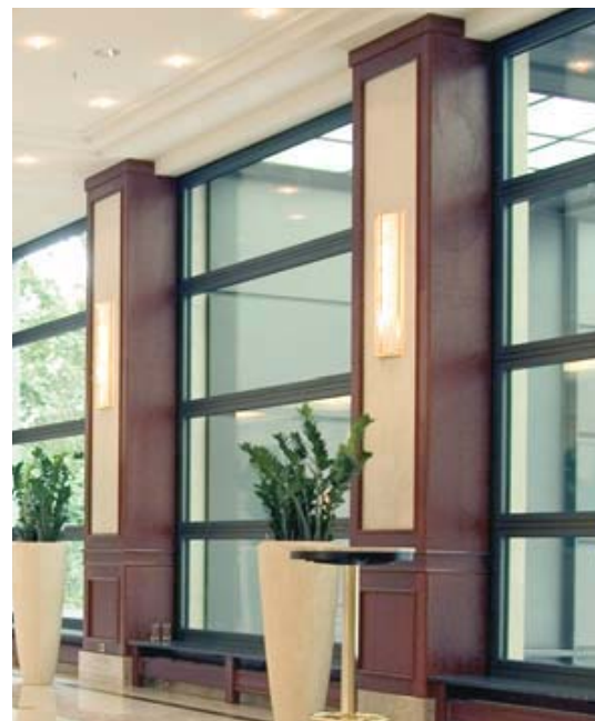
Four-light window units in hotel lobby
