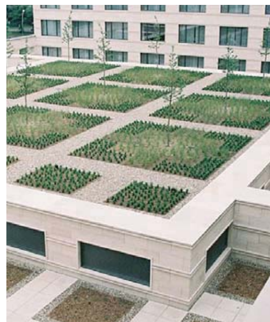
Raised roof area over Grand Ballroom with smoke vents
