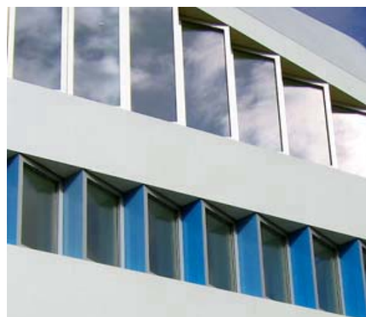
Top: The brilliant white-grey of the coated aluminium cassettes and sharp edges of the zigzagging windows set the ZVE apart from its surroundings; Bottom: Close-up of sawtooth windows
