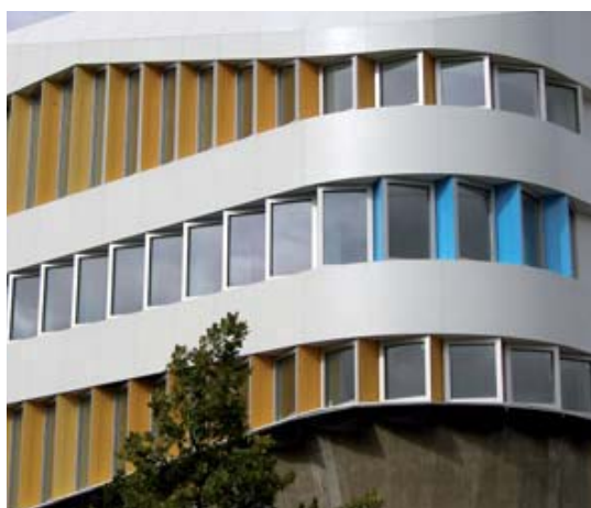
Top: The brilliant white-grey of the coated aluminium cassettes and sharp edges of the zigzagging windows set the ZVE apart from its surroundings; Bottom: Close-up of sawtooth windows
