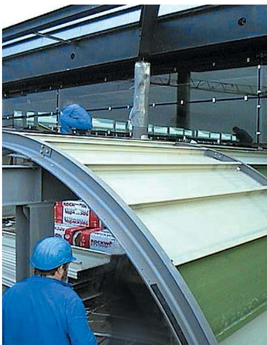
Installation of sheet-steel cassettes for administration block
