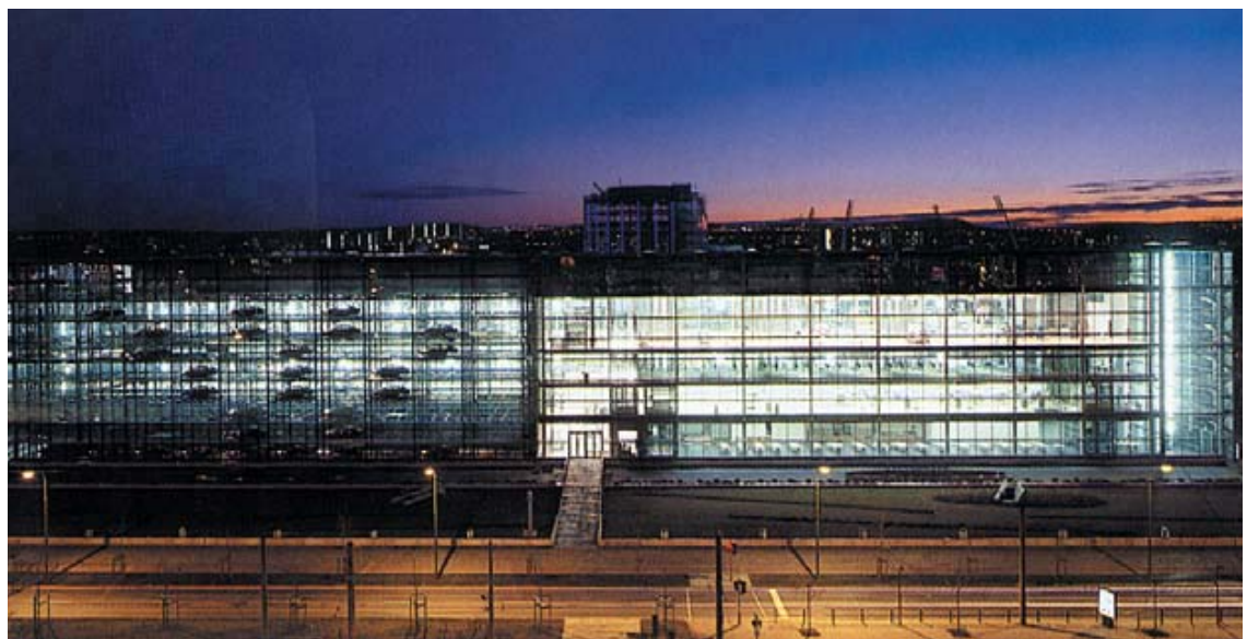
General view from north-east by night
