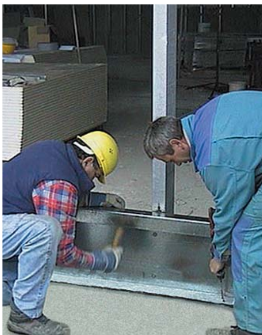
Installation of metal base for rooftop plantroom in VIP area
