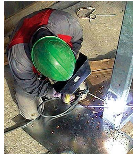
Welding works to steel mullions in VIP area
