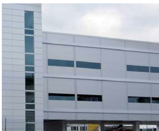
Front and rear view of passageway facades
