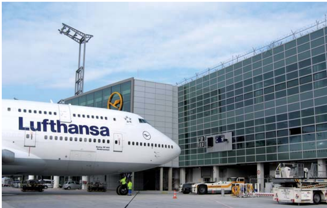
External view of a gate facade
