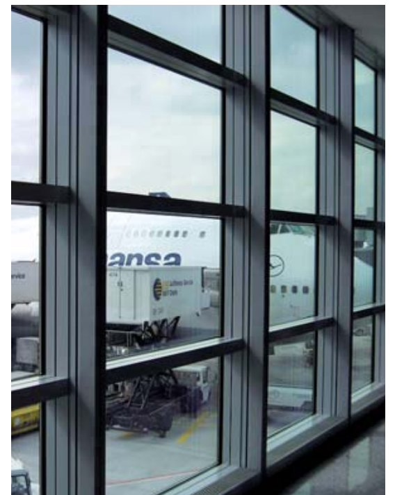
Internal view of a gate facade
