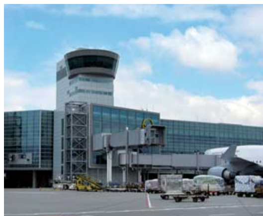
View of C/D pier facades from apron
