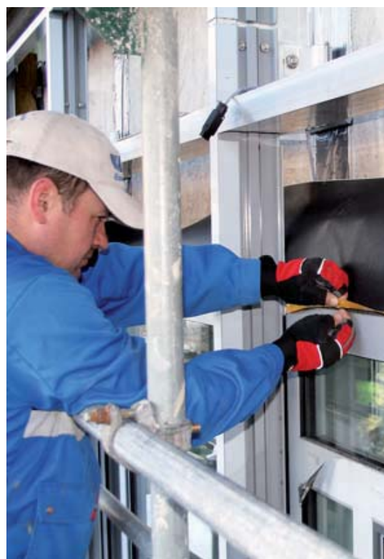
New window units are sealed (left) and old windows dismantled from inside building (right)
