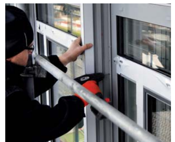
Top: Entire building wrapped in scaffolding prior to installation; Bottom: Fixing brackets mounted to structural fabric; new window units installed on inner face of vertical mullions
