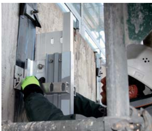
Top: Entire building wrapped in scaffolding prior to installation; Bottom: Fixing brackets mounted to structural fabric; new window units installed on inner face of vertical mullions
