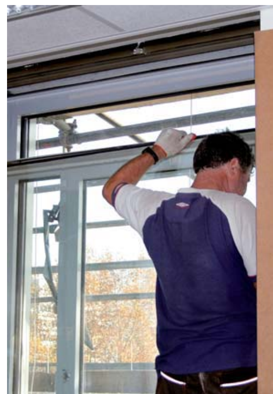
New window units are sealed (left) and old windows dismantled from inside building (right)
