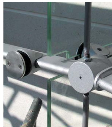
Detail view: nodes, glass clamps, transoms and tie rods
