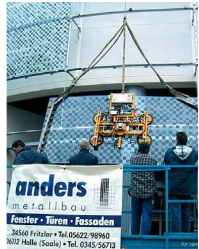
Installation of glazing with suction cup device
