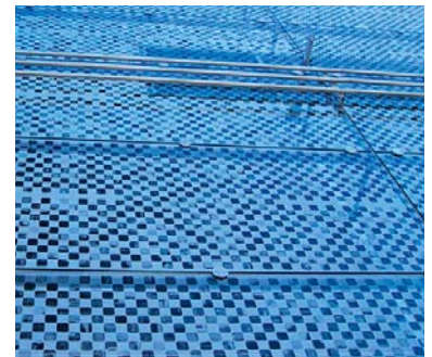
Half-tone screenprint techniques allowed photos to be displayed on facade
