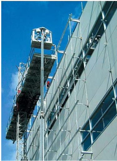
Erection of steelwork
